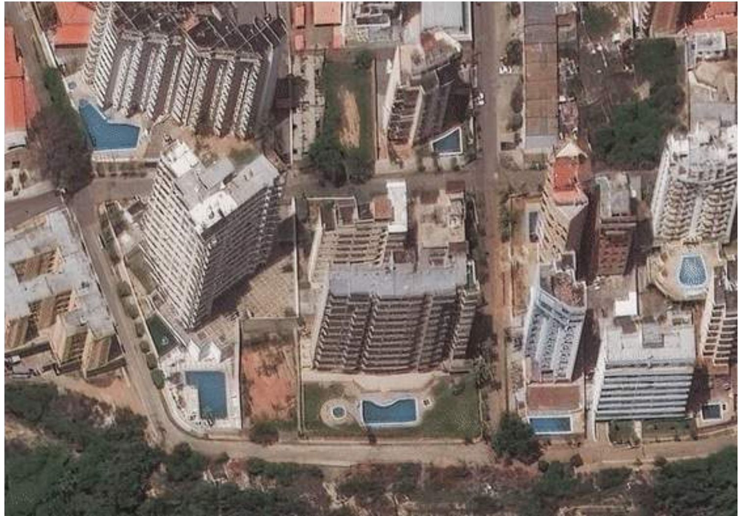
Apartment building in La Guaira, Venezuela, on June 22, and on June 25 2026 after the earthquakes. Satellite image ©2026 Vantor
